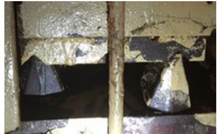
*Rockers not properly positioned
